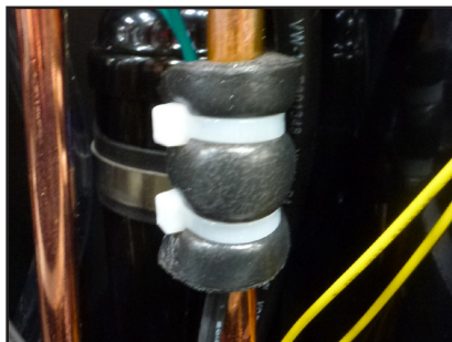
Figure 6: Thermistor attached to the refrigerant line.
